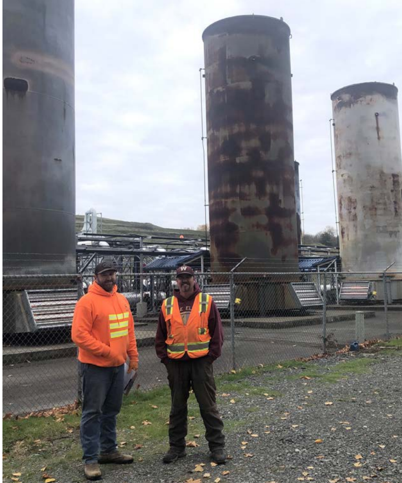
From left to right: Local 302 Landfill Gas Operators Rusty Korich and Rusty Bogart stand in front of the flares used to burn off methane gas. When waste is buried in the landfill it decomposes and produces methane gas. At Cedar Hills, a network of pipes capture that gas and route it to flares for destruction, or to an onsite renewable gas-to-energy facility operated by Bio Energy Washington (BEW) for processing. Some of the gas is converted to electricity for use on site by BEW, however most is cleaned of impurities and made into compressed natural gas and sold to Puget Sound Energy. King County is currently flaring the landfill gas as required by the environmental permits as BEW is not operating at this time.
