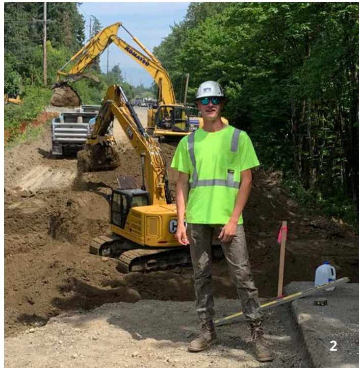
1. Ryan Mack rigging water line for the Judy Reservoir in Skagit County, working for Scarsella Brothers, Inc
