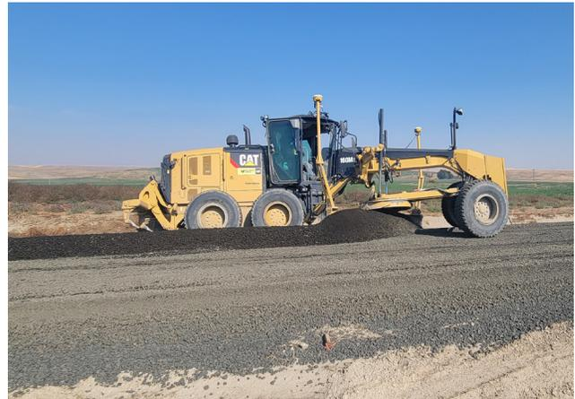
Operator Mark Thomas blading road for Apollo Inc. in a motor grader for the Highway 12 job
