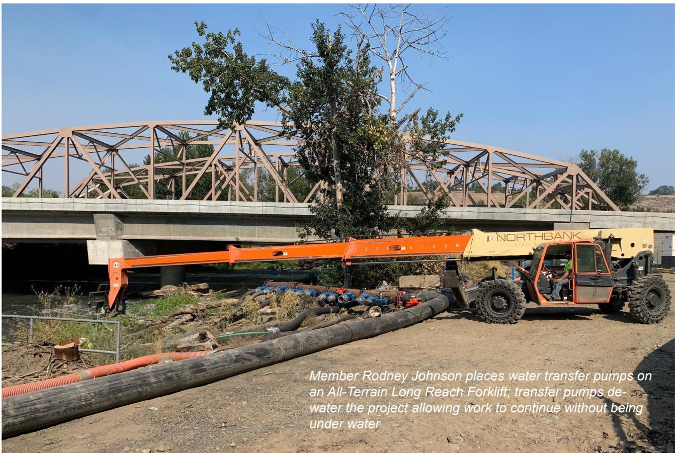
*Member Rodney Johnson places water transfer pumps on an All-Terrain Long Reach Forklift; transfer pumps de-water the project allowing work to continue without being under water*
