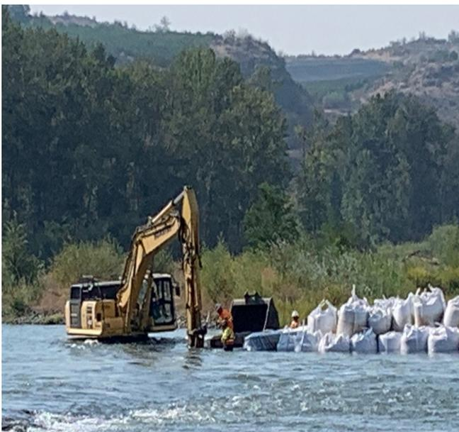
*Member Chris Clark runs the excavator and member Josh Thompson helps with placement of materials to divert the river so they can work in the main channel without water intrusion*
