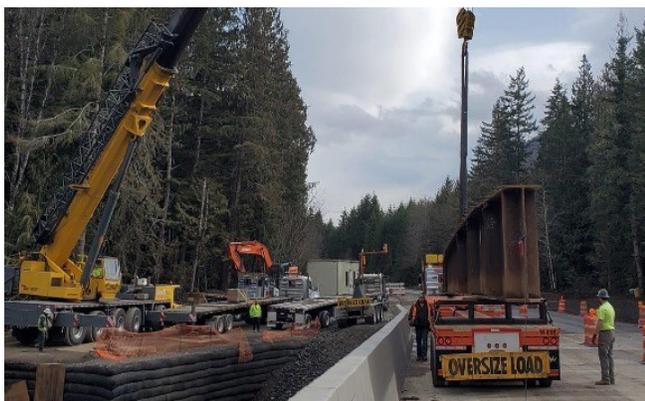
*Snell Crane Service removing the girders from the temporary bridge at the Indian Creek Project*
