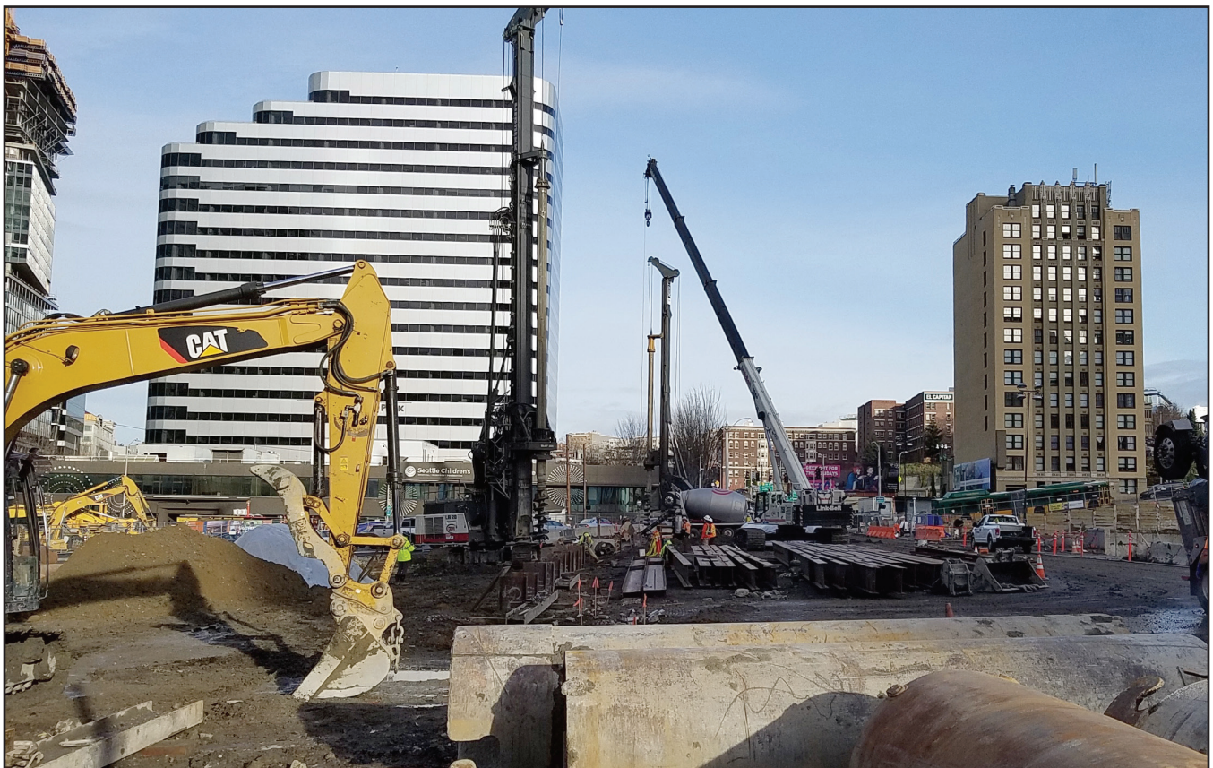
DBM Drilling at the Convention Center - Seattle, WA
