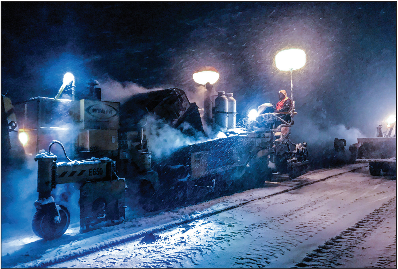
Pruhs Construction - Earthquake Repair on the Glenn Highway
