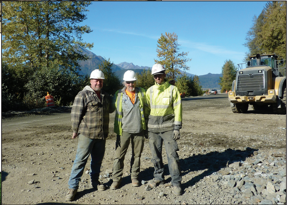
Crusher operators Shawn Lovell, Tim Ward, and Chris Downer working for Secon on the Haines Hwy phase 1 Project.
