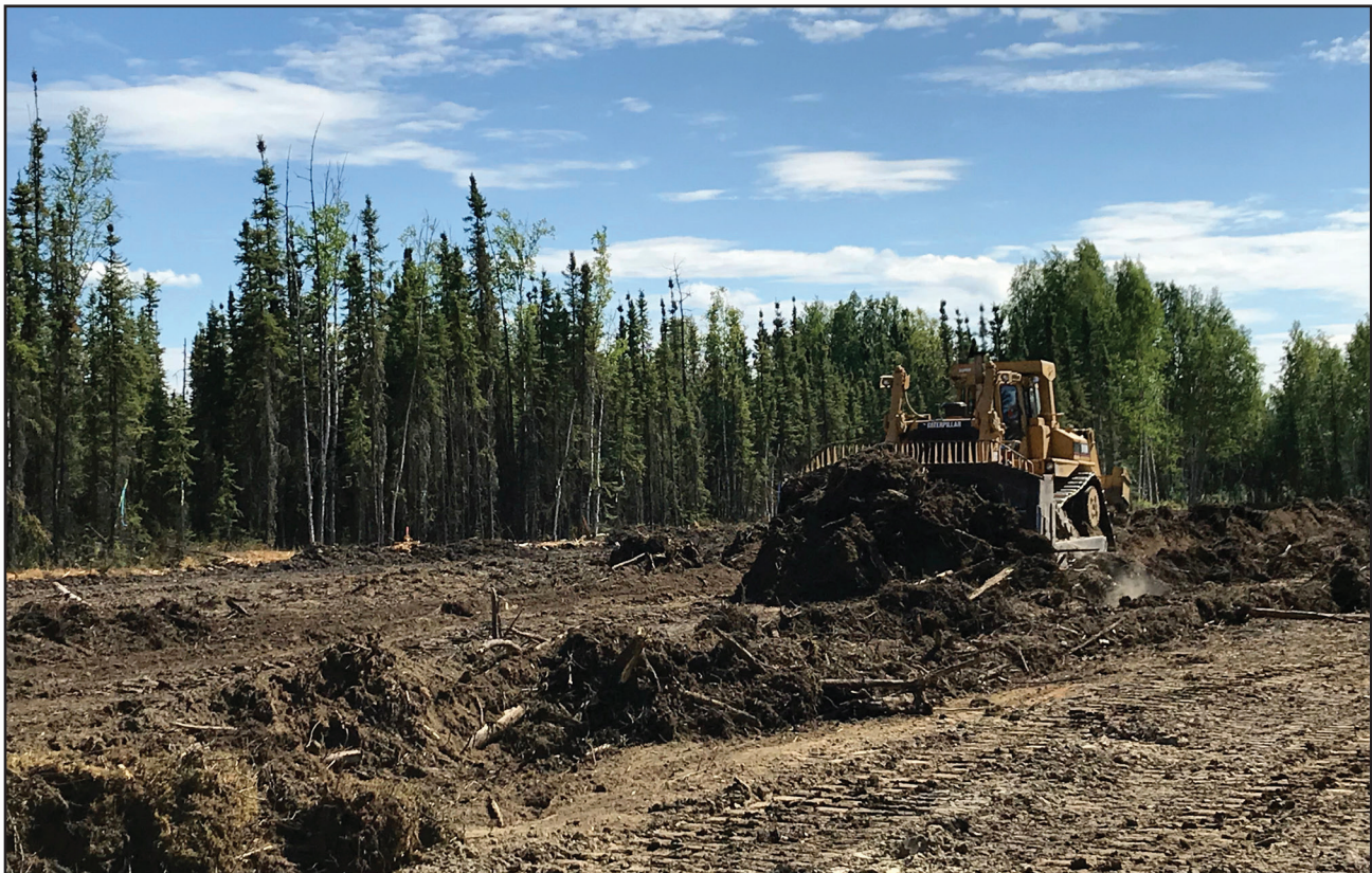
Eielson AFB Utililidoor Project-Mass Excavation, Inc
