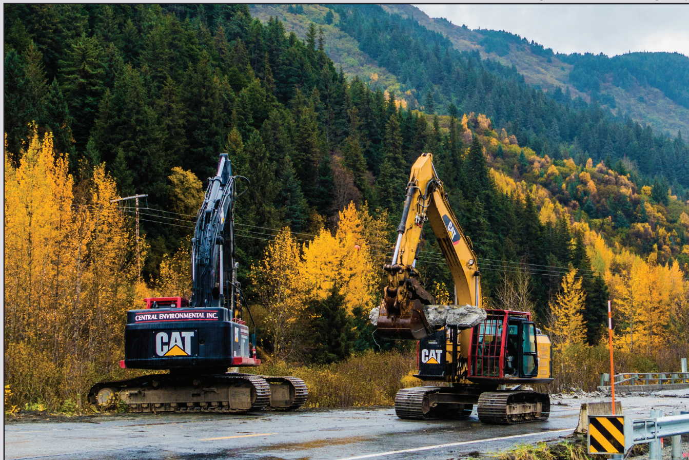
CEI working on the Seward Highway
