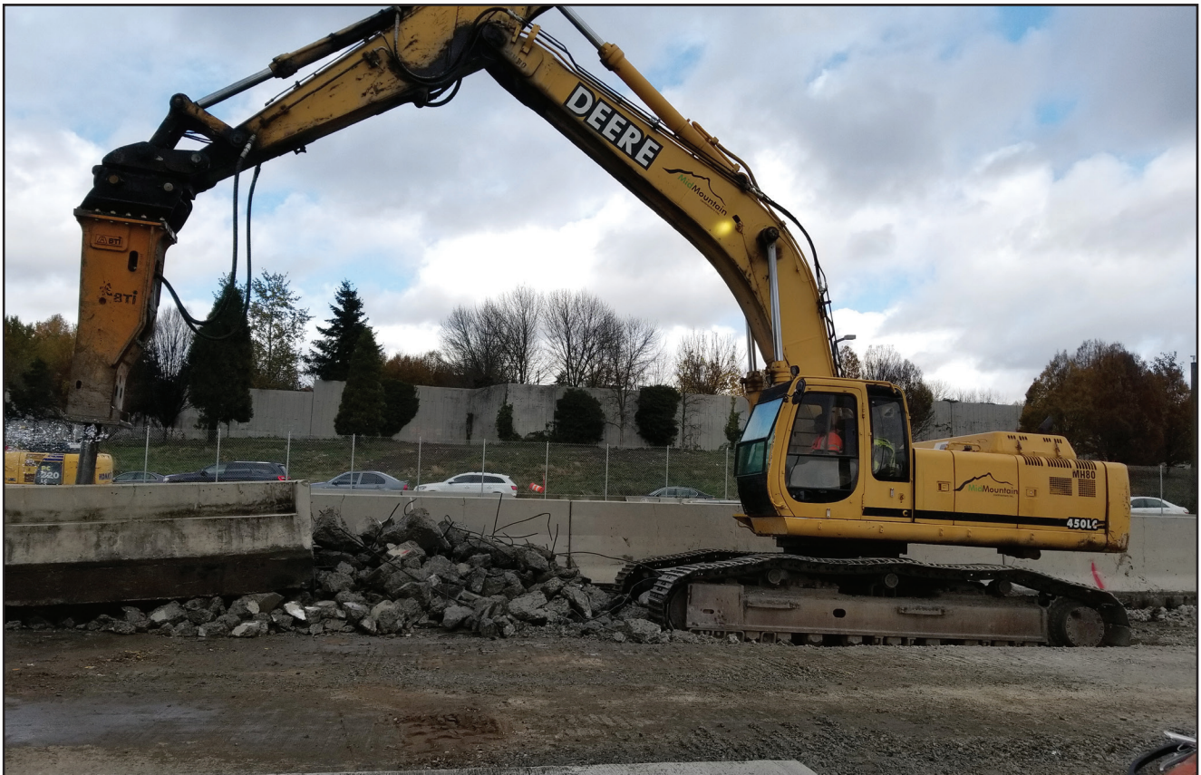
Sound Transit E 130 Project - Mid Mountain Apprentice Islynn Jackson
