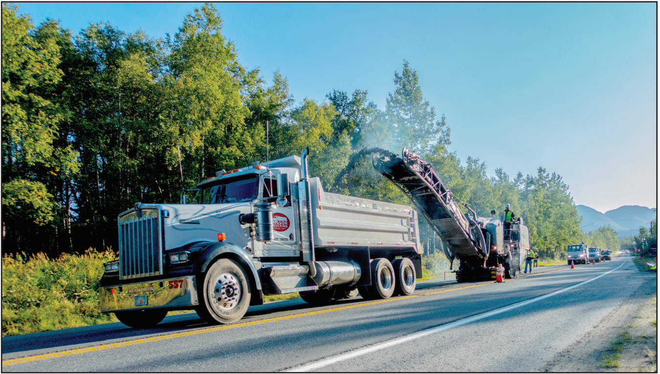
Granite Construction on Rabbit Creek Road
