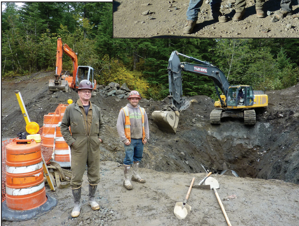
Operator Lynn Kirkham and Apprentice Jarett Thomas working for Coogan Construction
