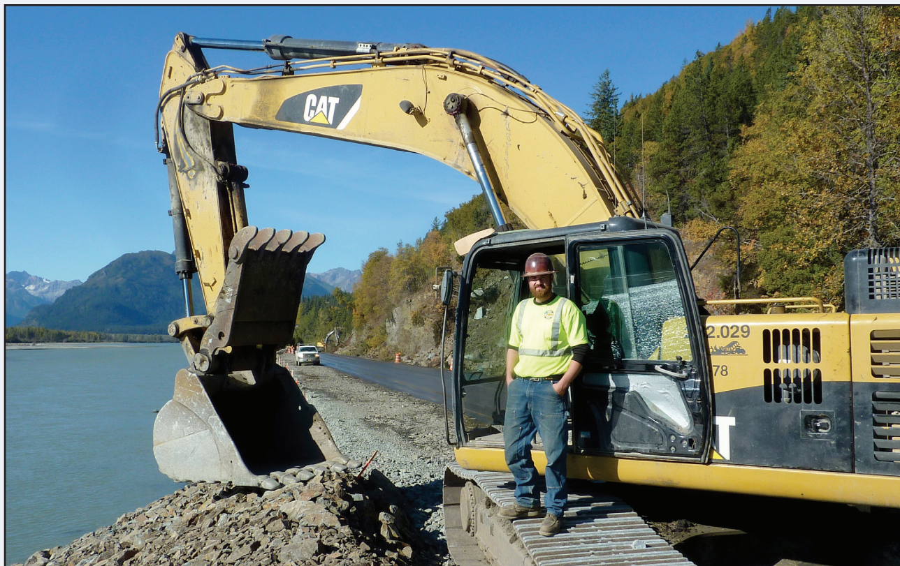
Nate Narum operating excavator for Secon Construction Haines Hwy Project.
