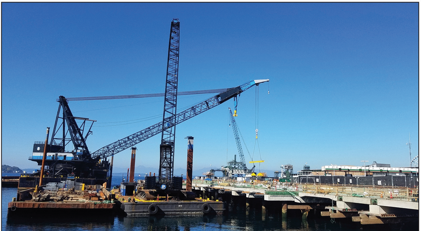
Pacific Lifter - Coleman Dock Project
