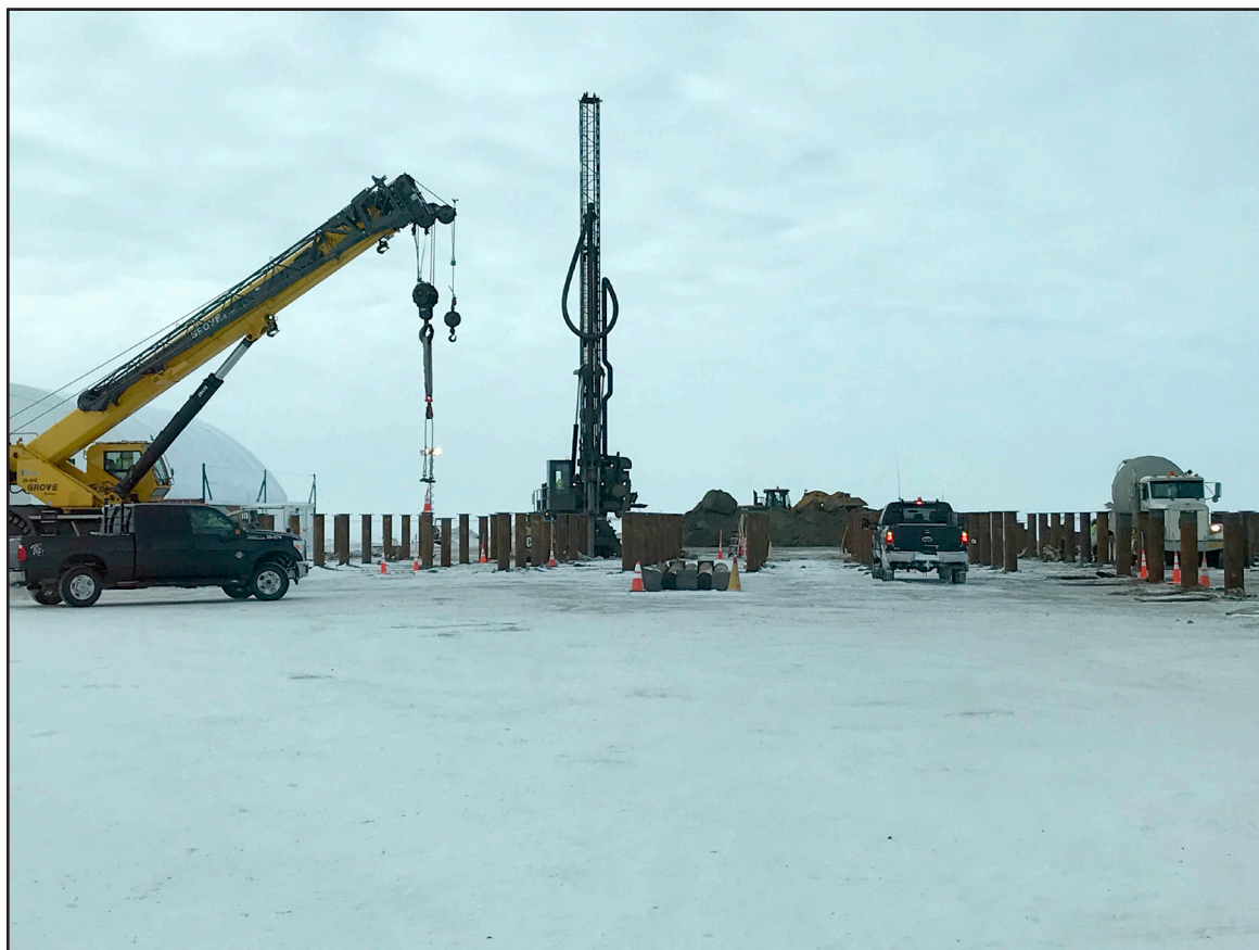
Daryl Gibson operating a Watson Drill for AFC on Moose Pad for setting piles.
