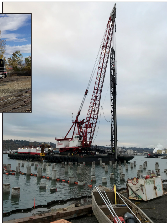
Manson DB Scandia driving 24" solid concrete piles at terminal 4 - Joel Condos -Operator and Pat Sullivan -Deck Engineer.
