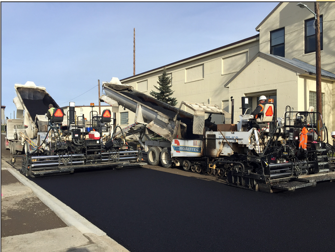
Bob White and Dale Schram both running topside on two pavers running side by side to eliminate any joint density requirements.
