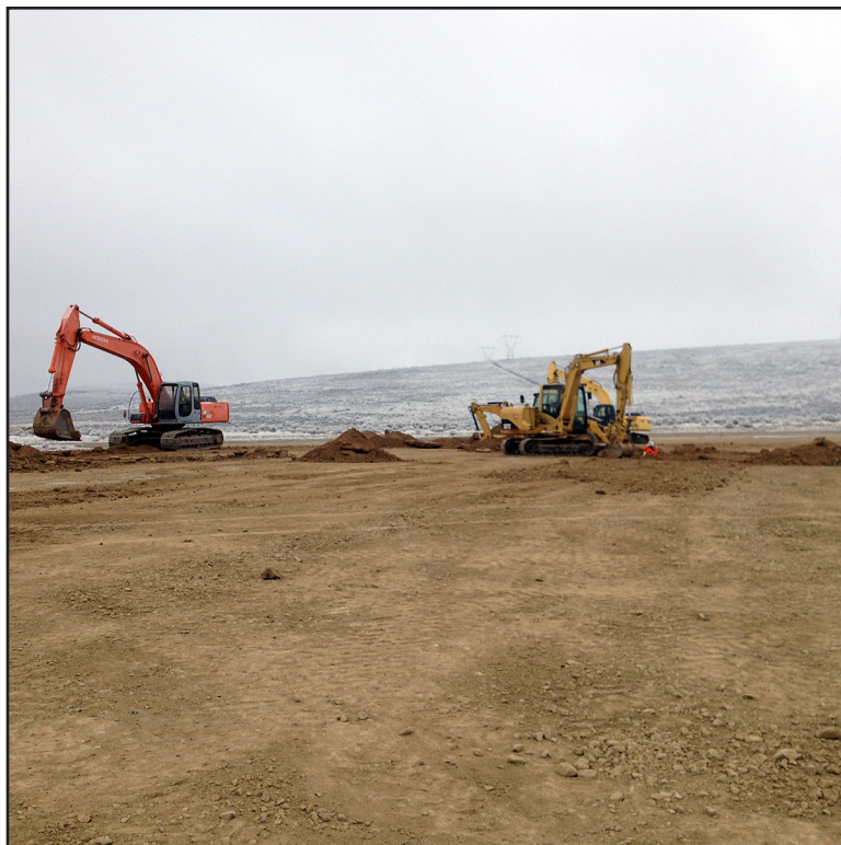
Excavators chunking their way through the frozen top levels
